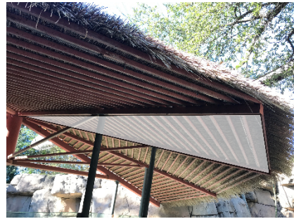
Photo SEQ Photo \* ARABIC \r 1 1 - Closeup of the penguin exhibit roof, highlighting one of the triangles that make up the roof. PC: Jonathan Edduid
